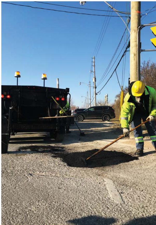
Municipal road maintenance staff are working around the clock to keep roads safe and accessible for those delivering essential services. Photo: City of Toronto
