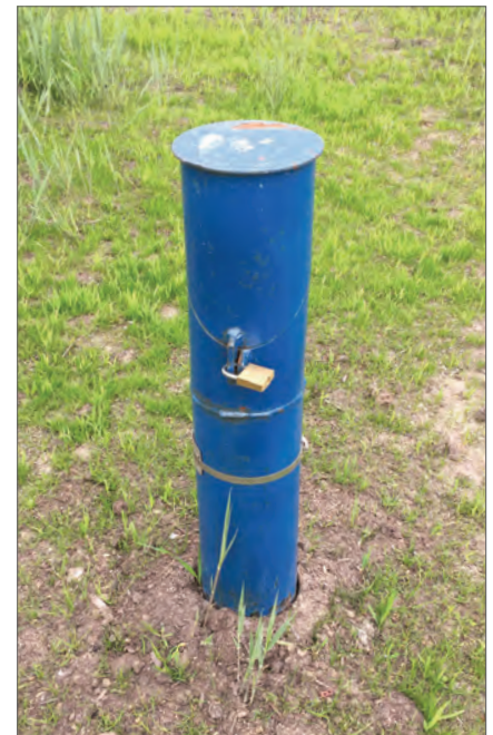
Example of a groundwater monitoring well
