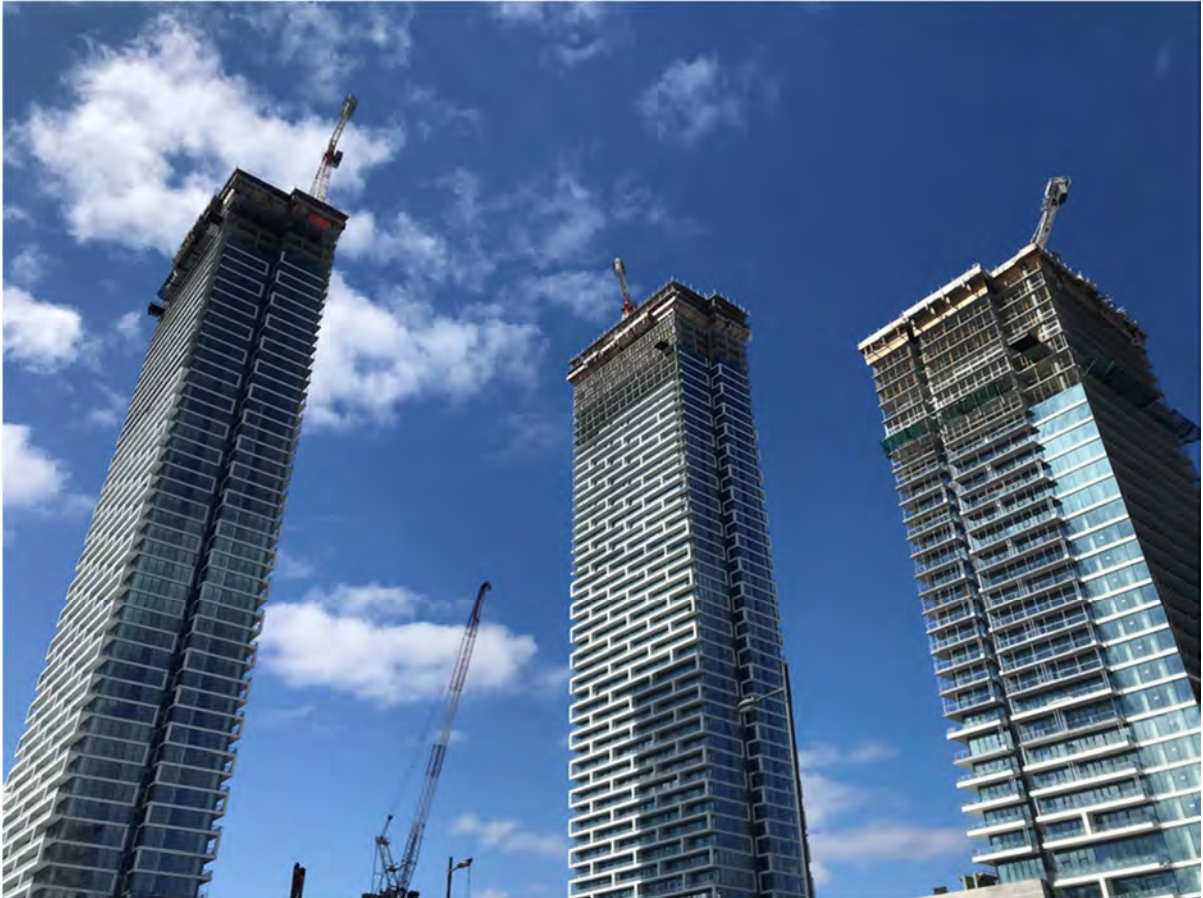
Figure 5 Buildings under construction at the Vaughan Metropolitan Centre
