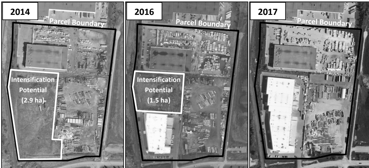
Image Location: 2190 Teston Road, Maple Employment Area, Vaughan Source: York Region Planning and Economic Development, March 2018
