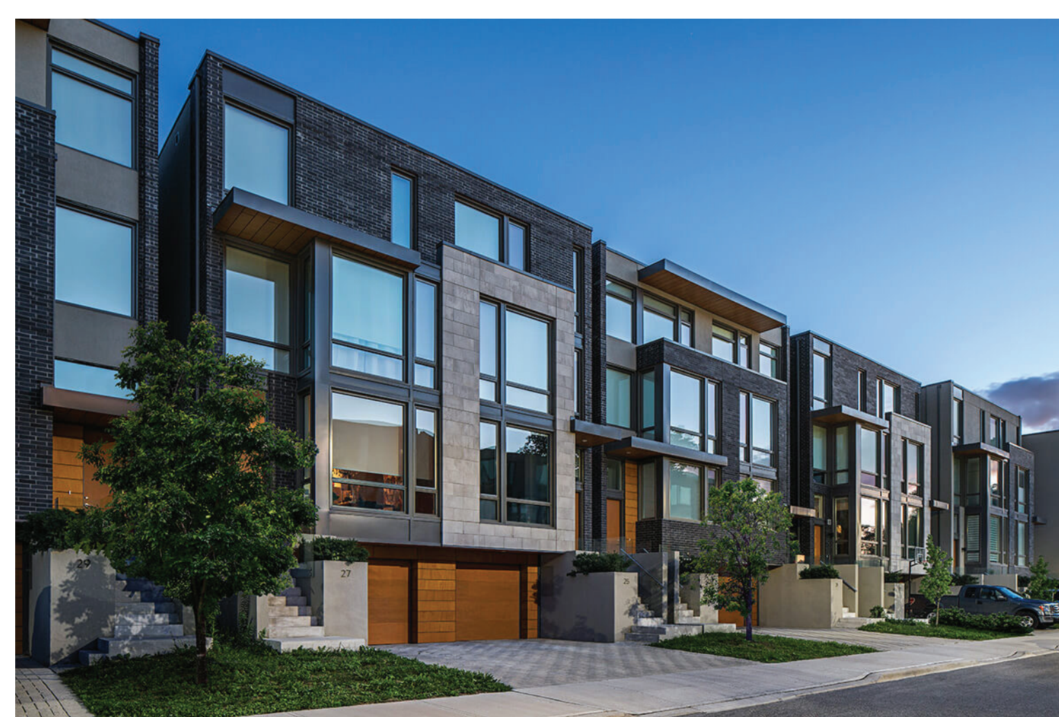
Edgewood, Image Credit - TACT Architecture
