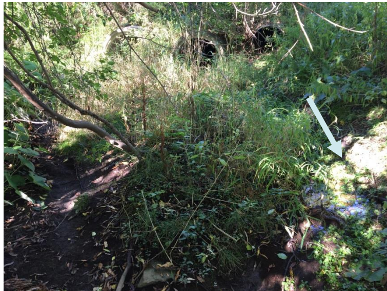
Photo 6: Outlet of multiple-barrel crossing under GO Transit rail line
