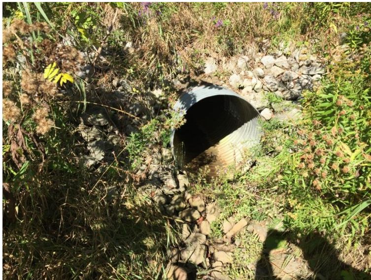
Photo 8: Outlet of culvert under Nokiidaa Bike Trail
