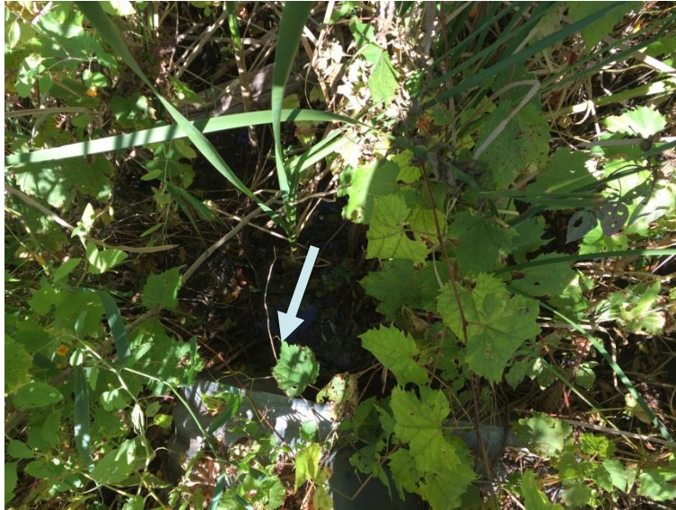
Photo 2: Entrance of culvert under Main Street North By-pass
