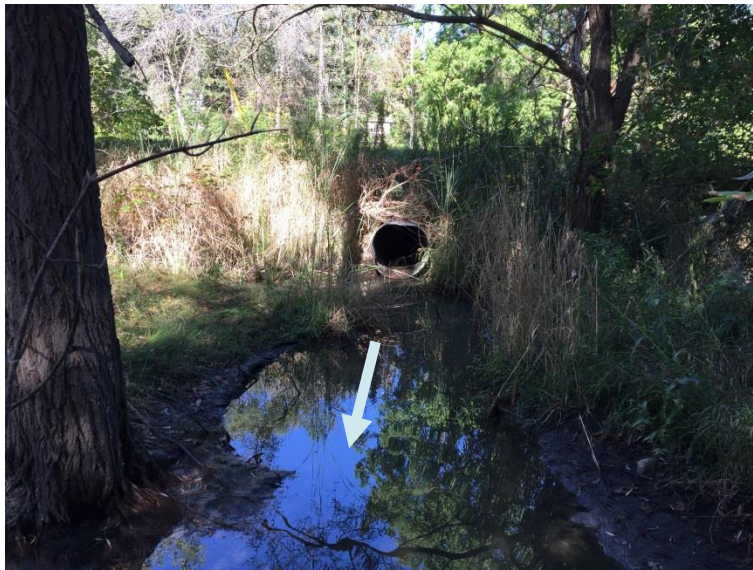
Photo 3: Outlet of culvert under Main Street North By-pass
