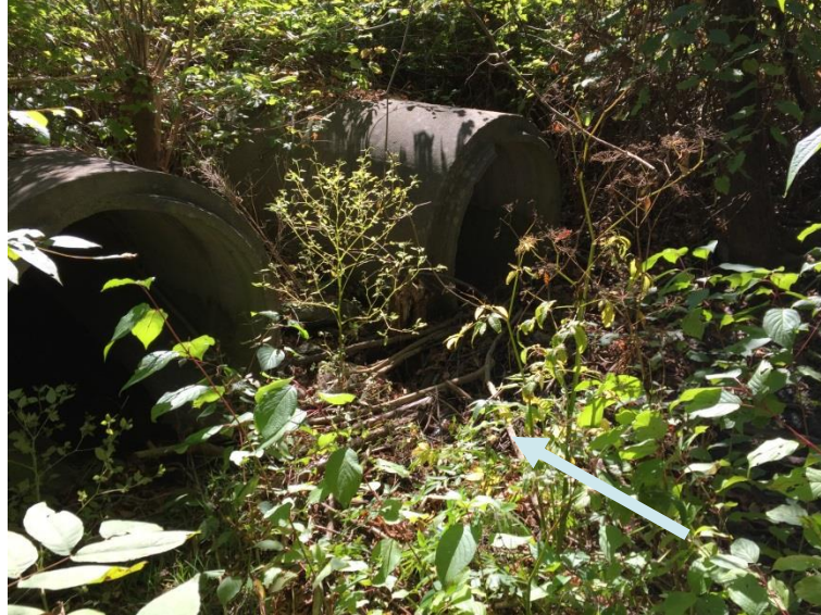
Photo 5: Entrance to concrete pipe culverts under GO Transit rail line
