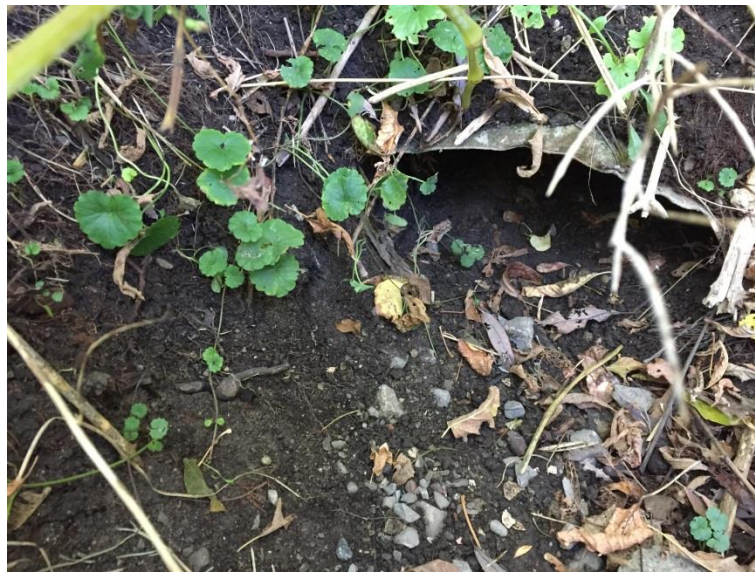
Photo 1: Outlet of culvert under roadway at No 194 Old Main Street
