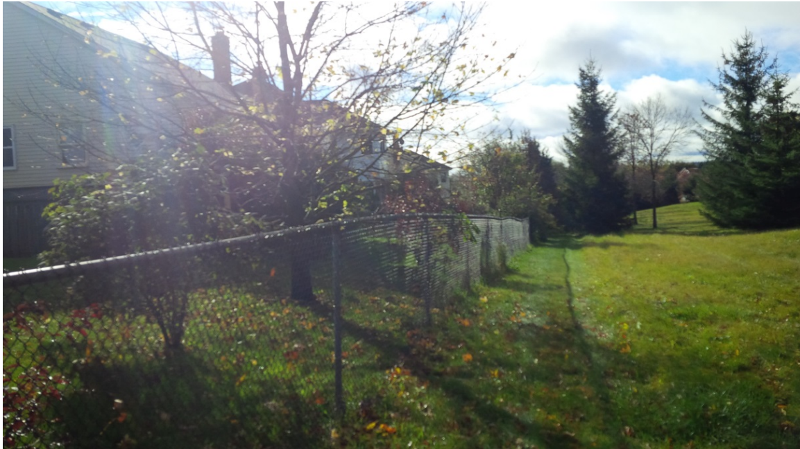
Figure 24: Existing Conditions along Section 2D
