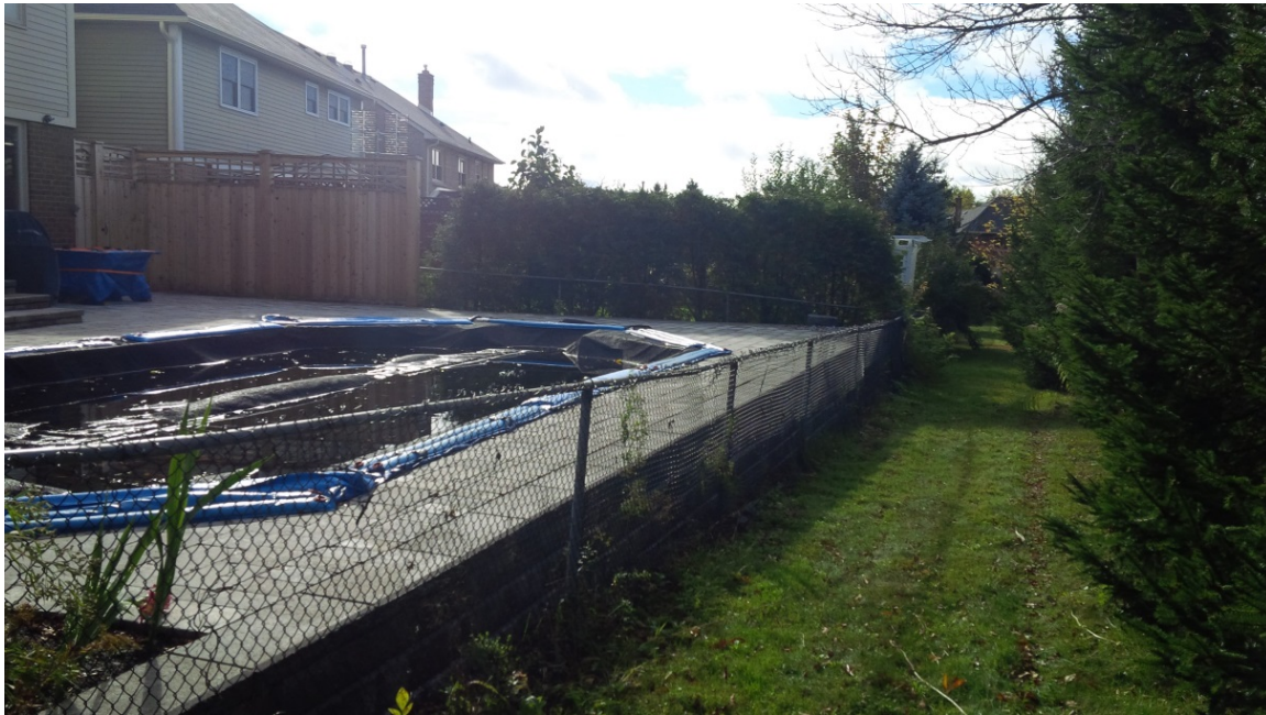
Figure 23: Existing Conditions along Section 2D
